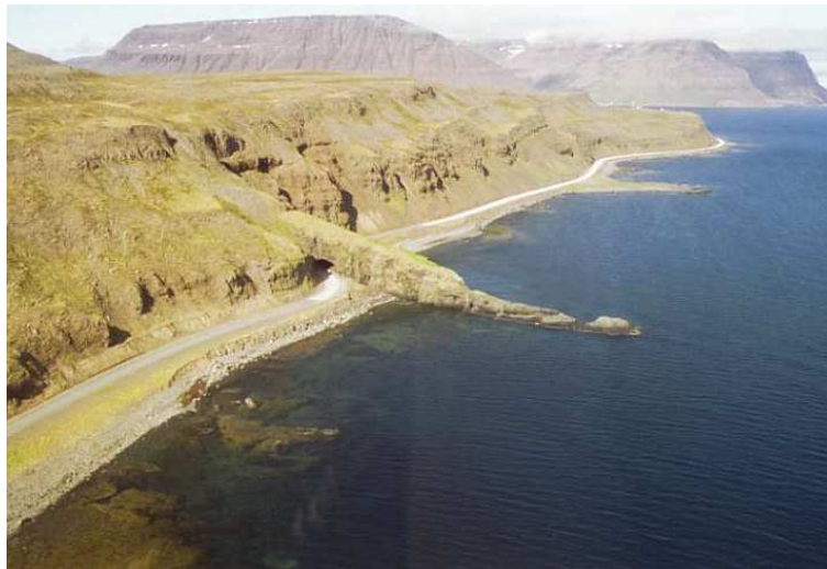
Figure 4-1. First tunneling project in Iceland, a road tunnel through Arnarneshamar finished in 1949 [Guðmundsson 1999].
