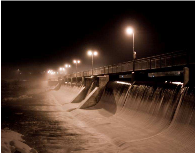
Figure 3-1. Hydropower plant at Elliðaá [Sigurðardóttir, 2008].
