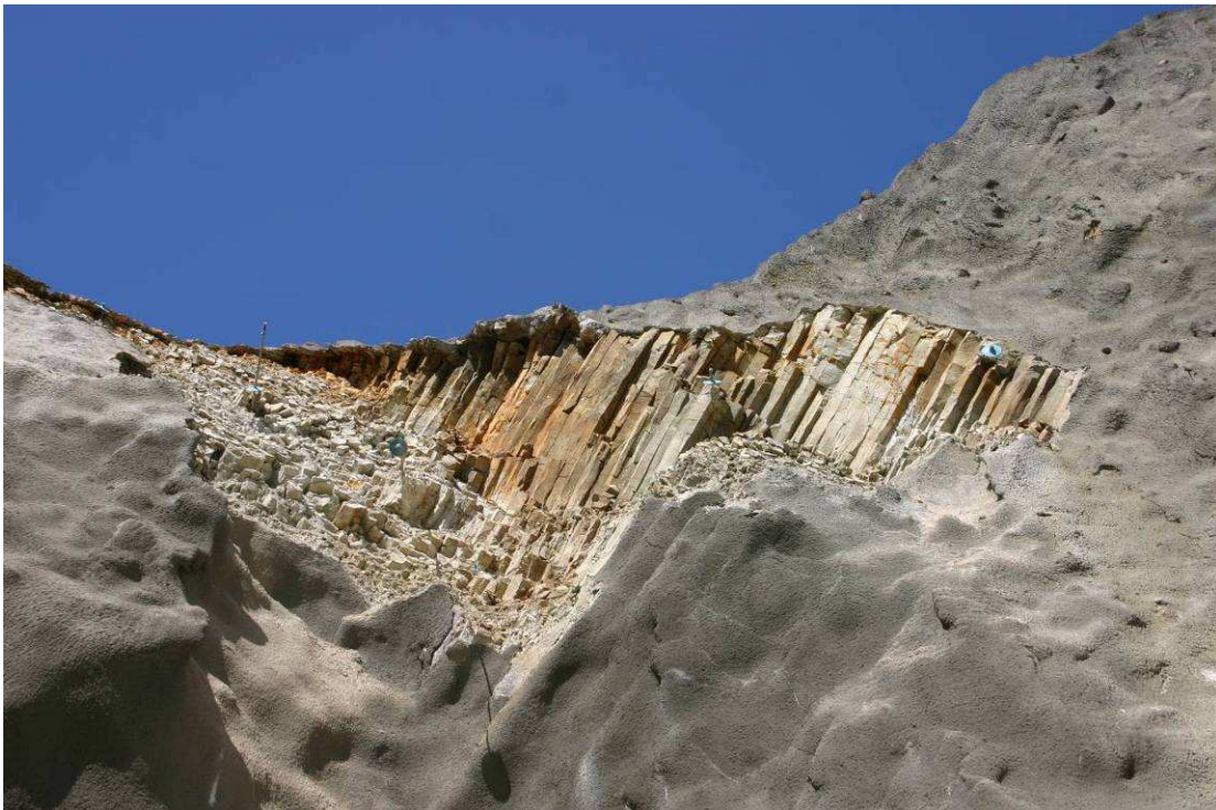
Figure 9-7. Excavation at Búðarháls Power Station foundation, note the small columnar joints, sprayed concrete and rockbolts [Gunnarsson photo, 2009].
