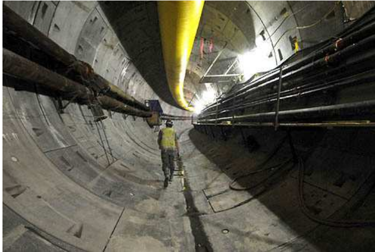
Figure 8-4. Pre-cast concrete support sections [Post-Gazette, 2008].
