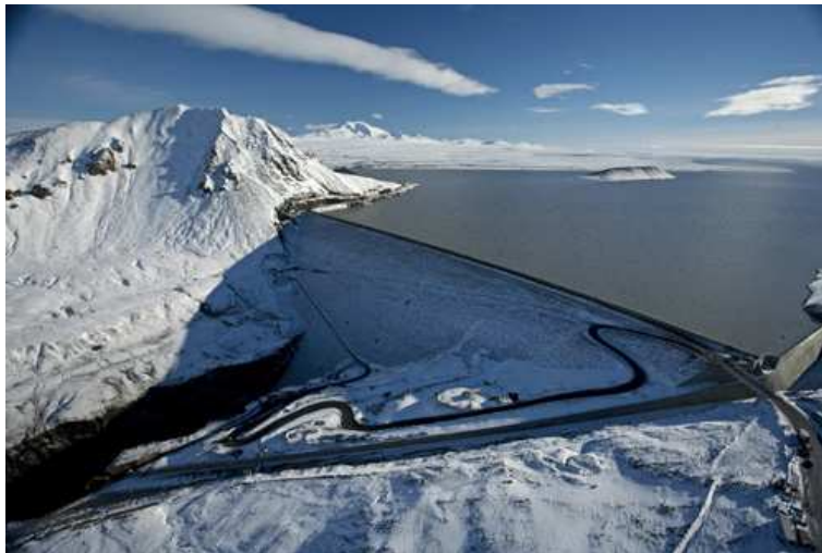
Figure 3-2. Kárahnjúkar hydropower dam [National geographic, 2009].
